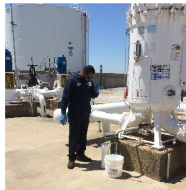
Figure 27. Fuel storage quality control.
