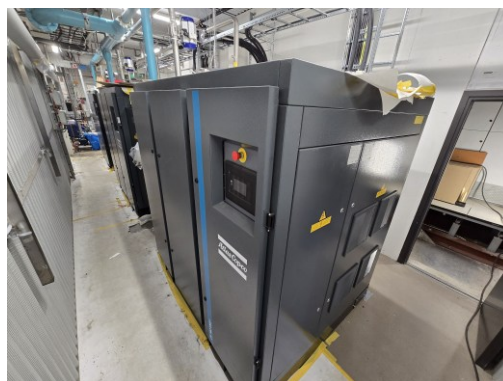
Figure 3. The new oil-free compressors were delivered in December 2024 and during the last year the installation including electrical supply, piping for compressed air and cooling water, has been finalized. The door opening to the right connects the compressor room with the switchgear central. To reduce electrical interferences, the separating wall is made of seam welded aluminum.
